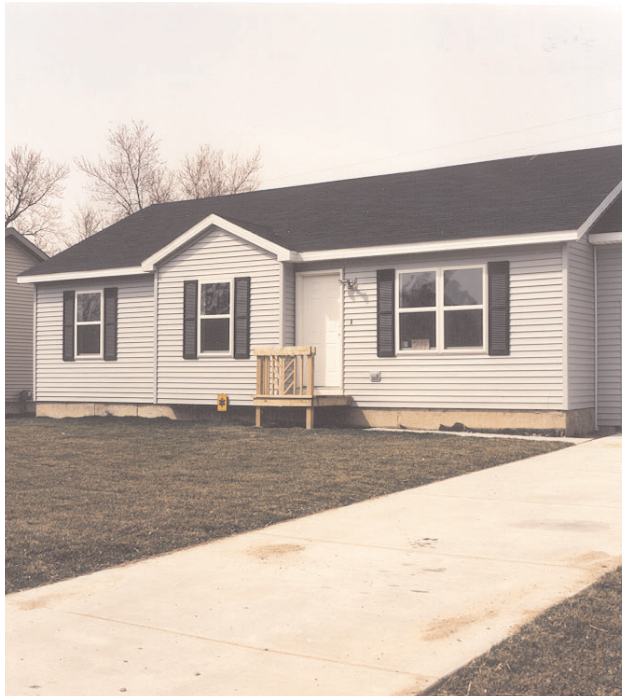
Single-story modulars fit into this neighborhood of eclectic home styles (courtesy, Venture, Inc.).
